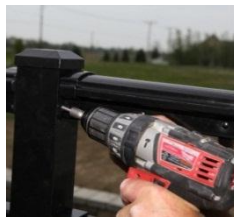
Installation Spindle – is screwed to post; best option when no angles are involved.
