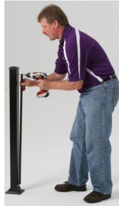
Installation Spindle – is screwed to post; best option when no angles are involved.
